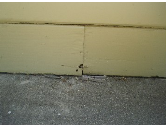
Gap in wood siding, side of house near laundry room. Repair.
